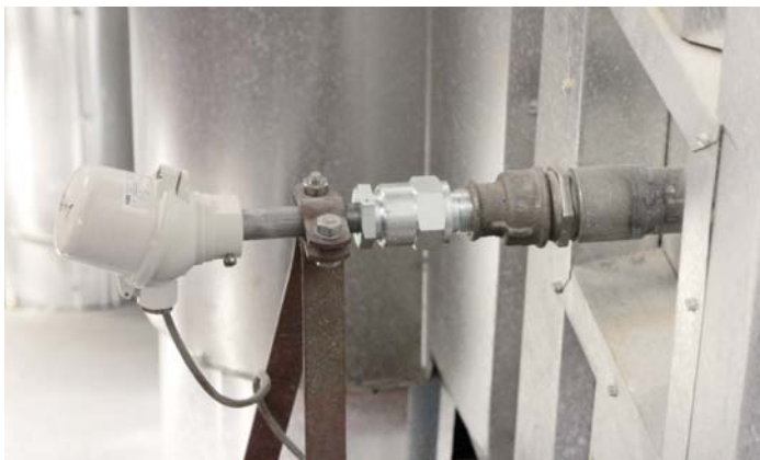
ABB high temperature sensor installed in a kiln
